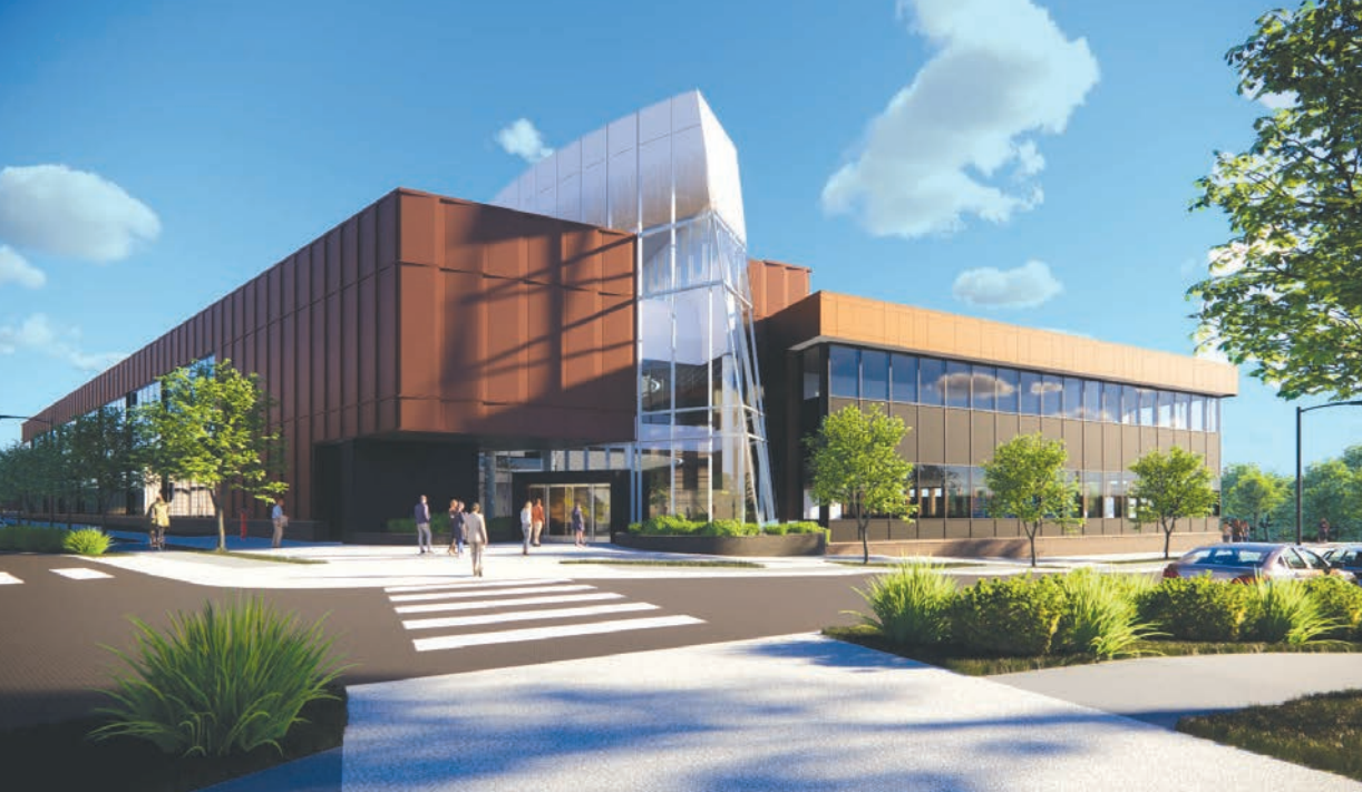
Pitt breaks ground for its BioForge facility at Hazelwood Green this spring.
